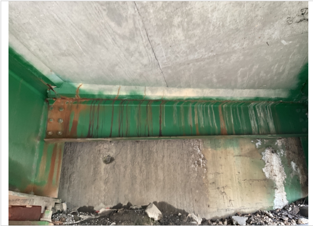
Span 1 diaphragm A corrosion
