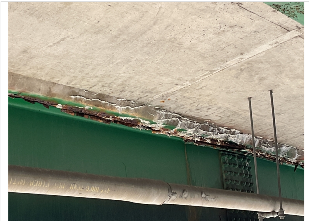
Span 3 Girder E top flange corrosion with eff
