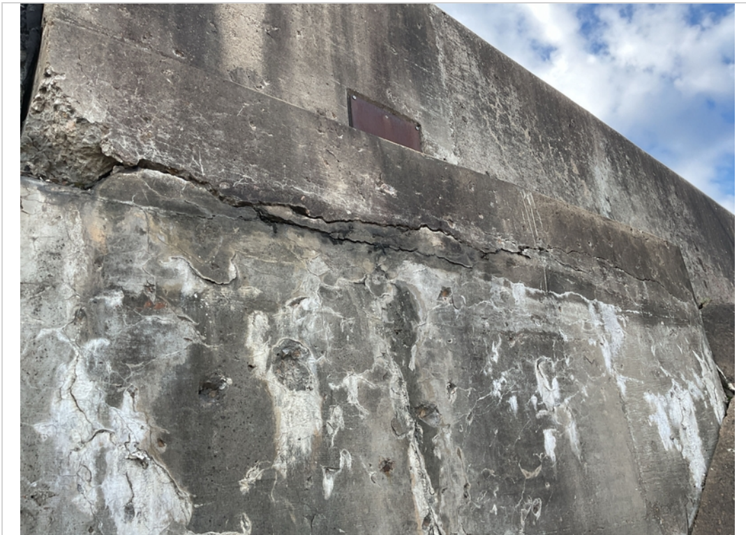
Abut 1 left wing open cracks hvy eff
