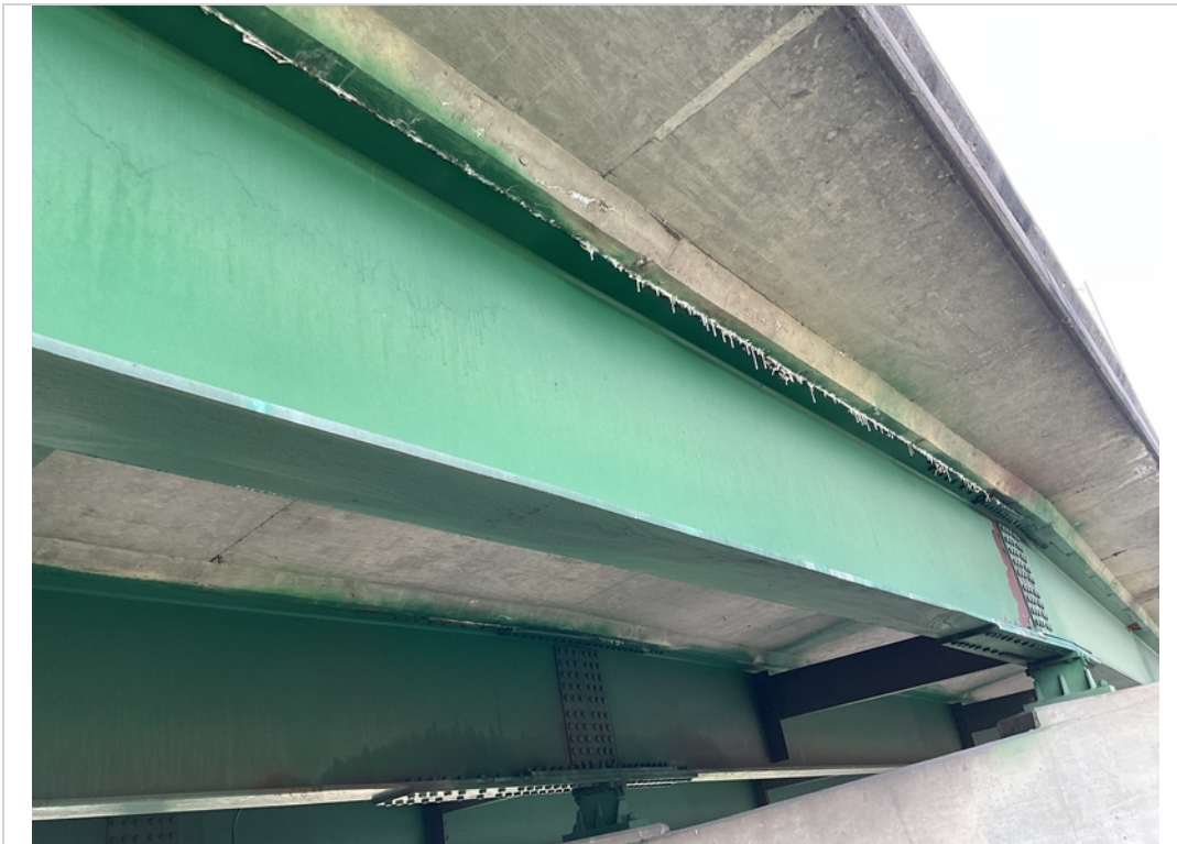
Span 3 Girder A top flange corrosion with eff
