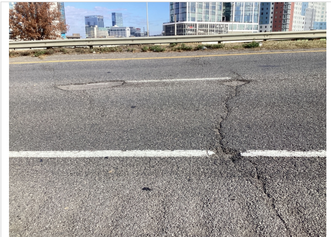
B approach pavement potholes
