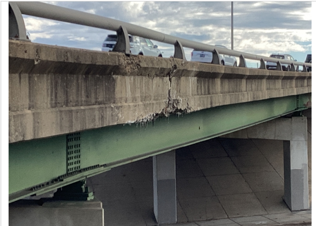
Span 2 parapet scale
