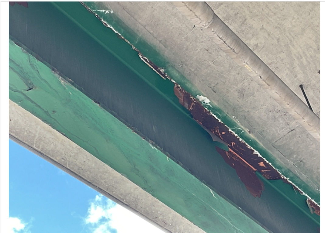
Span 2 Girder E top flange corrosion with eff
