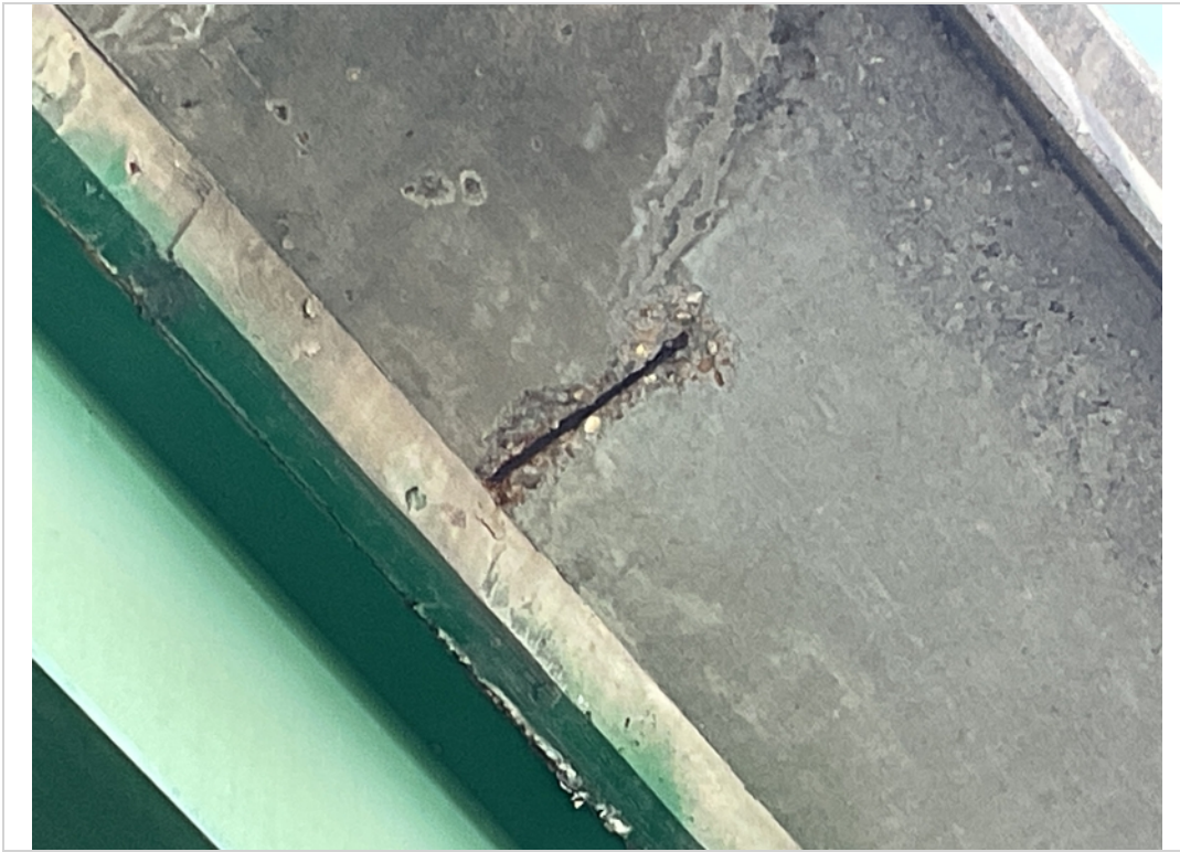
Overhang span 2 left side spall with exp steel
