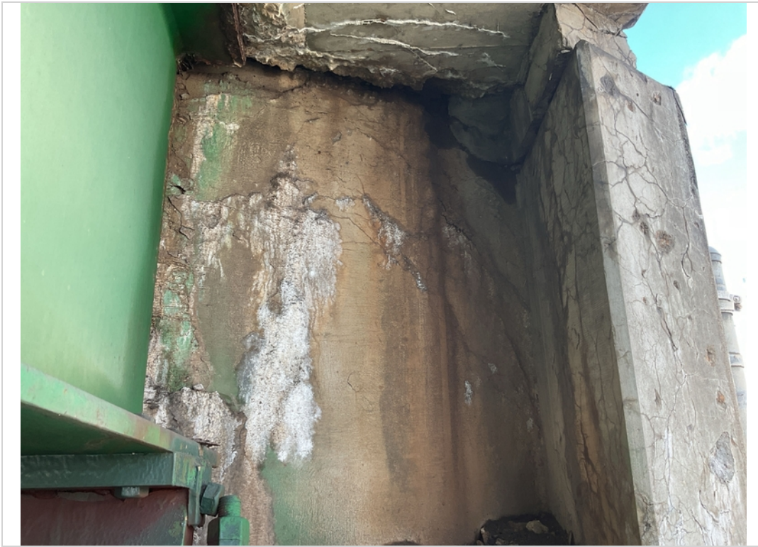
Abut 1 map cracks hvy eff
