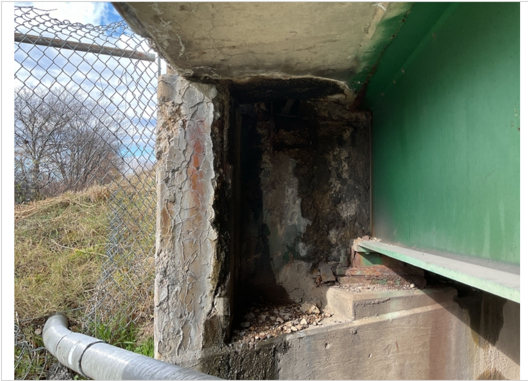
Abut 1 right wing map cracks
