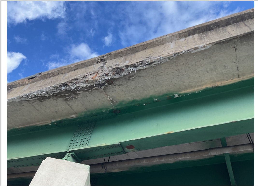
Overhang span 2 right side scale with eff
