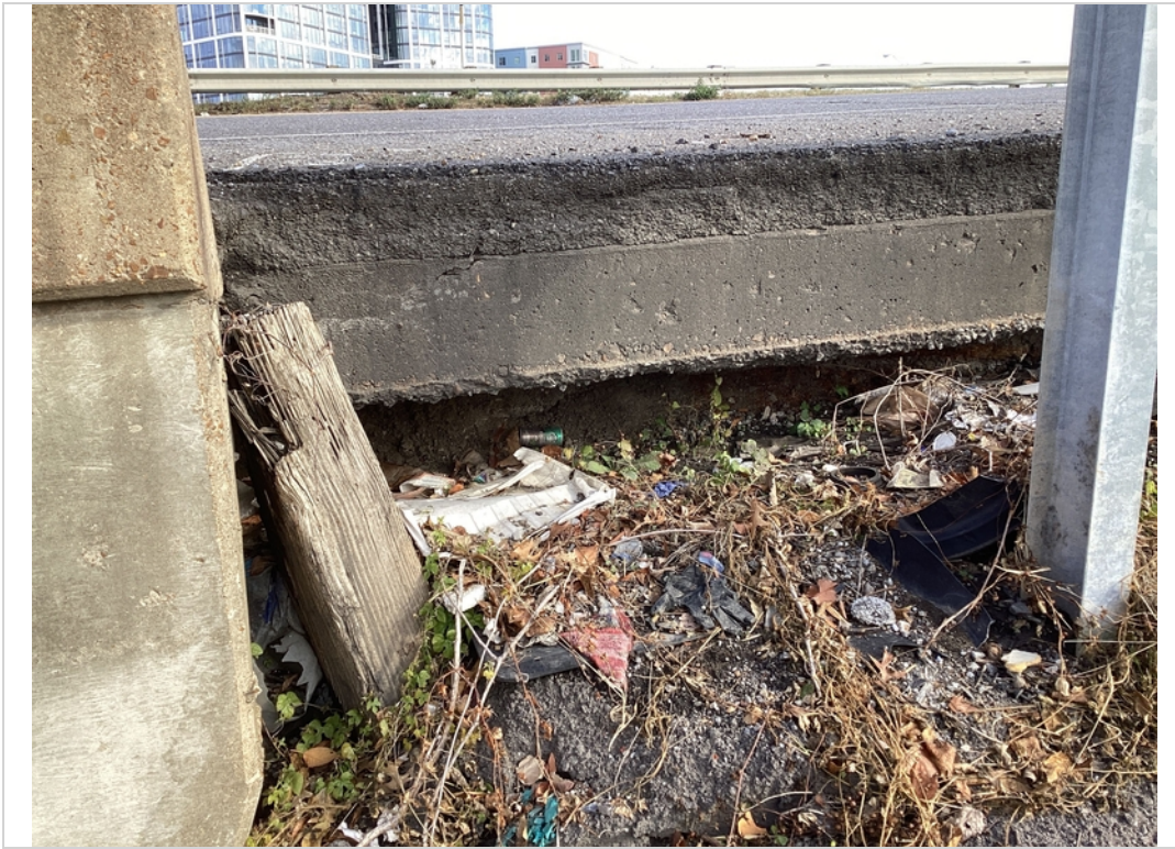
B approach heavy erosion
