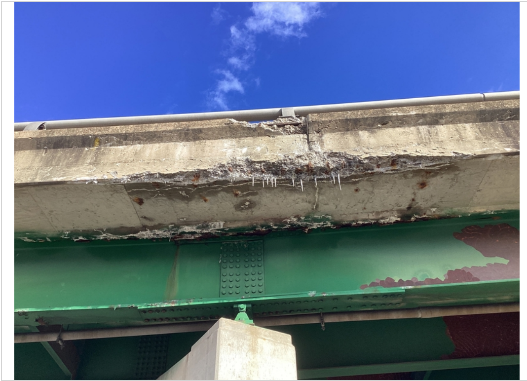
Parapet right span 3 heavy scale with exposed steel
