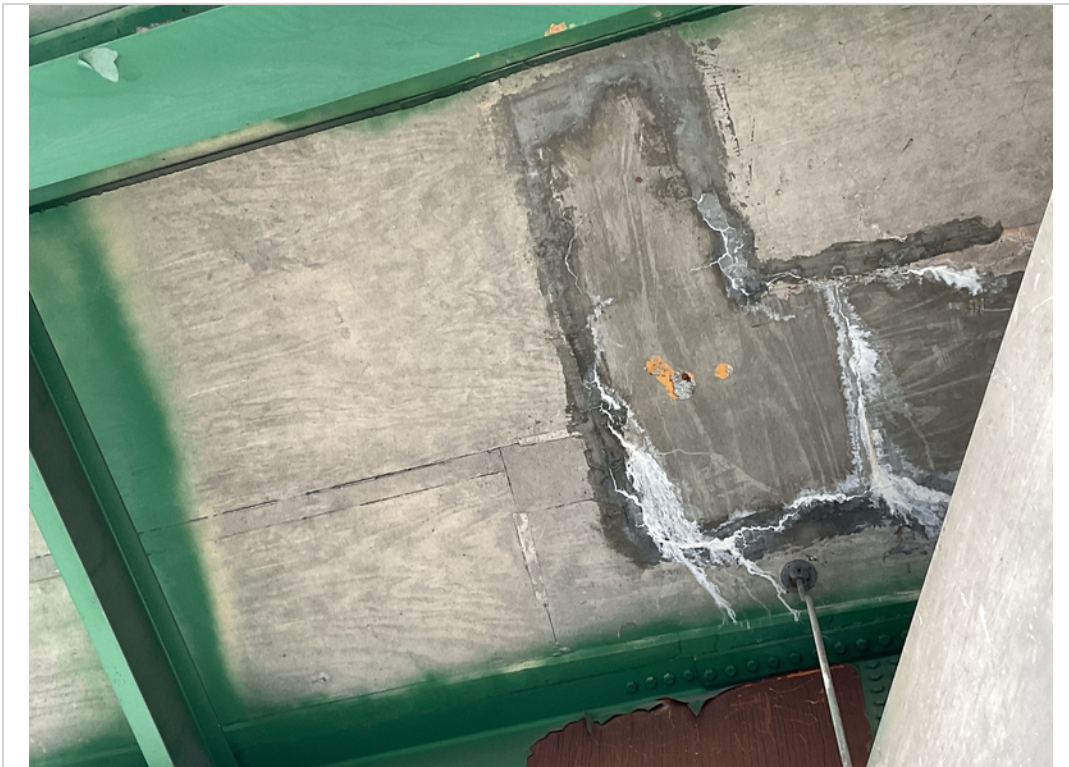
Span 2 bay B failing patch with eff
