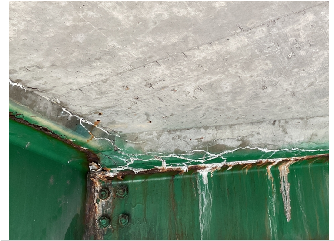
Span 1 bay D map cracks with eff
