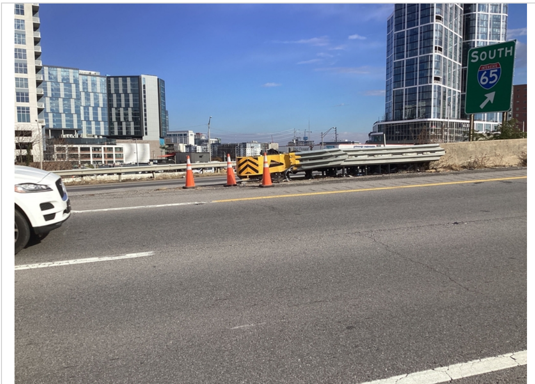
A approach end terminal impact damage
