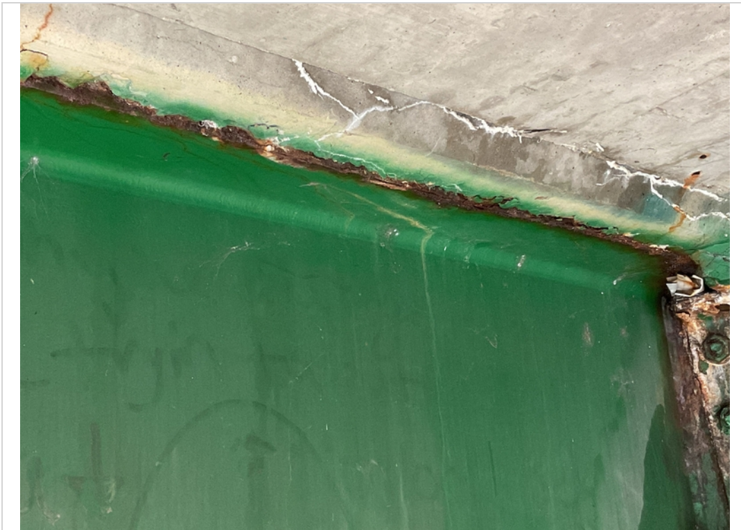
Span 1 Girder E top flange corrosion
