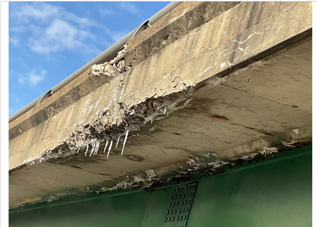
Overhang span 3 right side delam with eff
