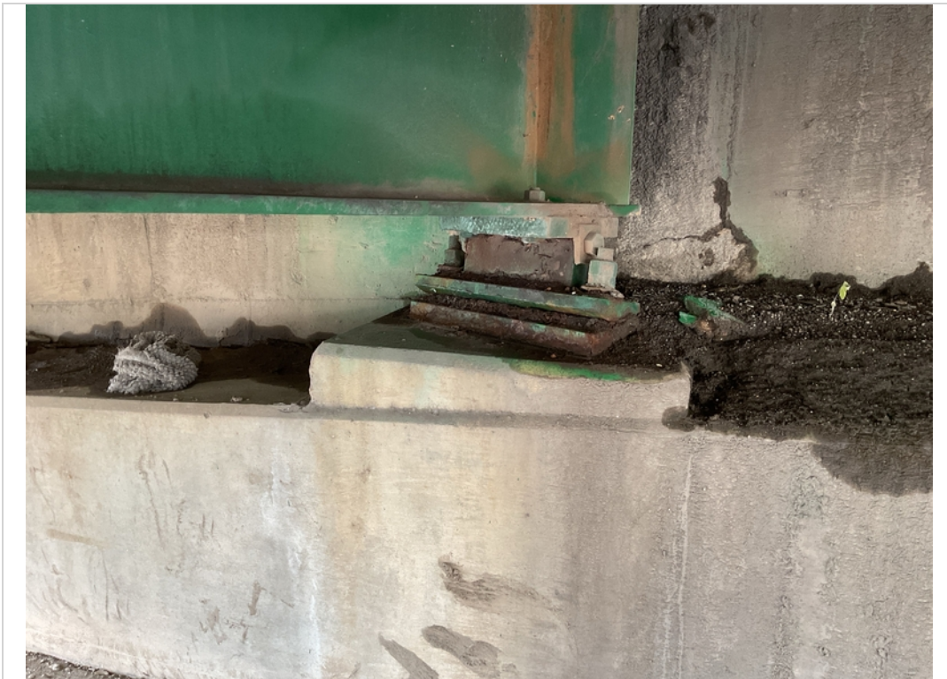
Abut 1 bearing D loose anchorage moderate corrosion
