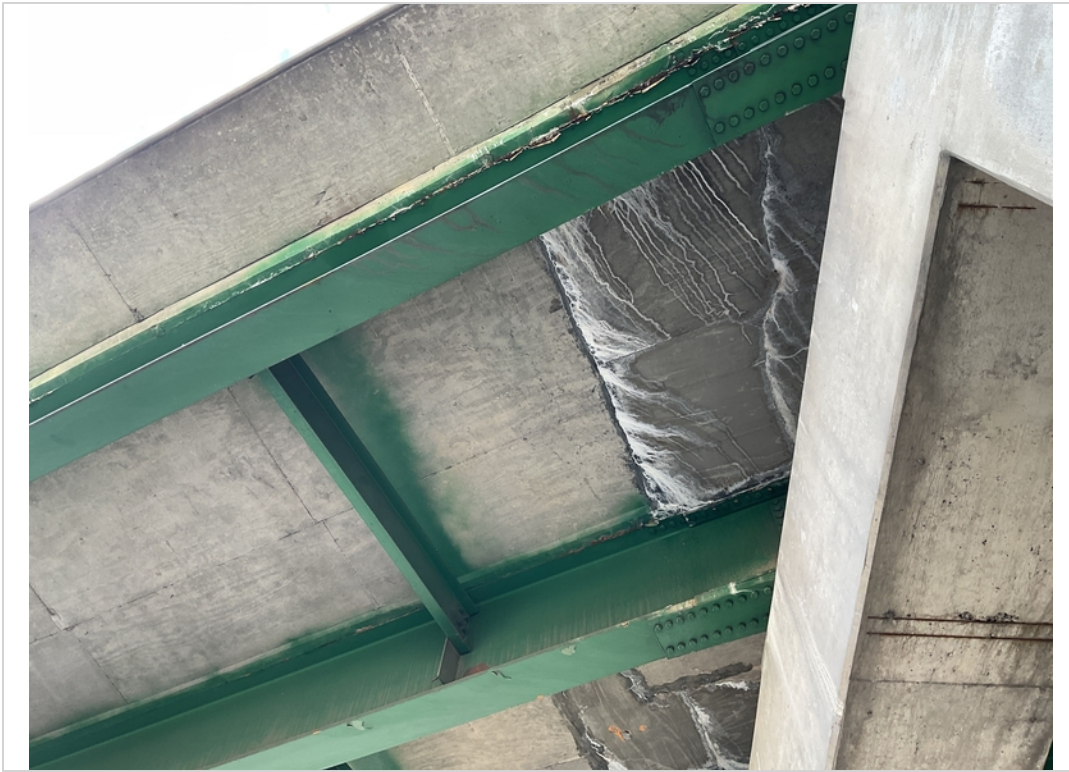
Span 2 bay A failing patch will eff
