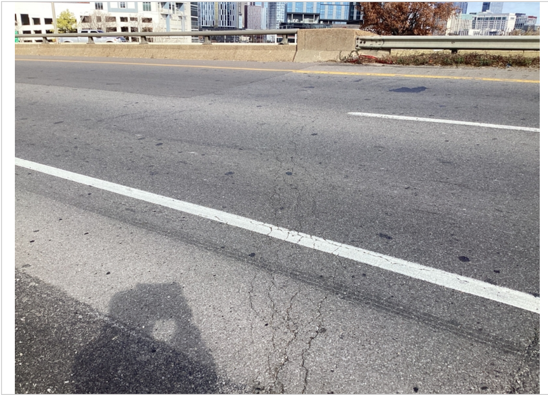
Span 3 map cracks
