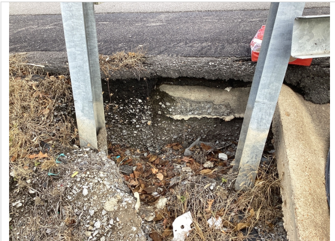
A approach right erosion
