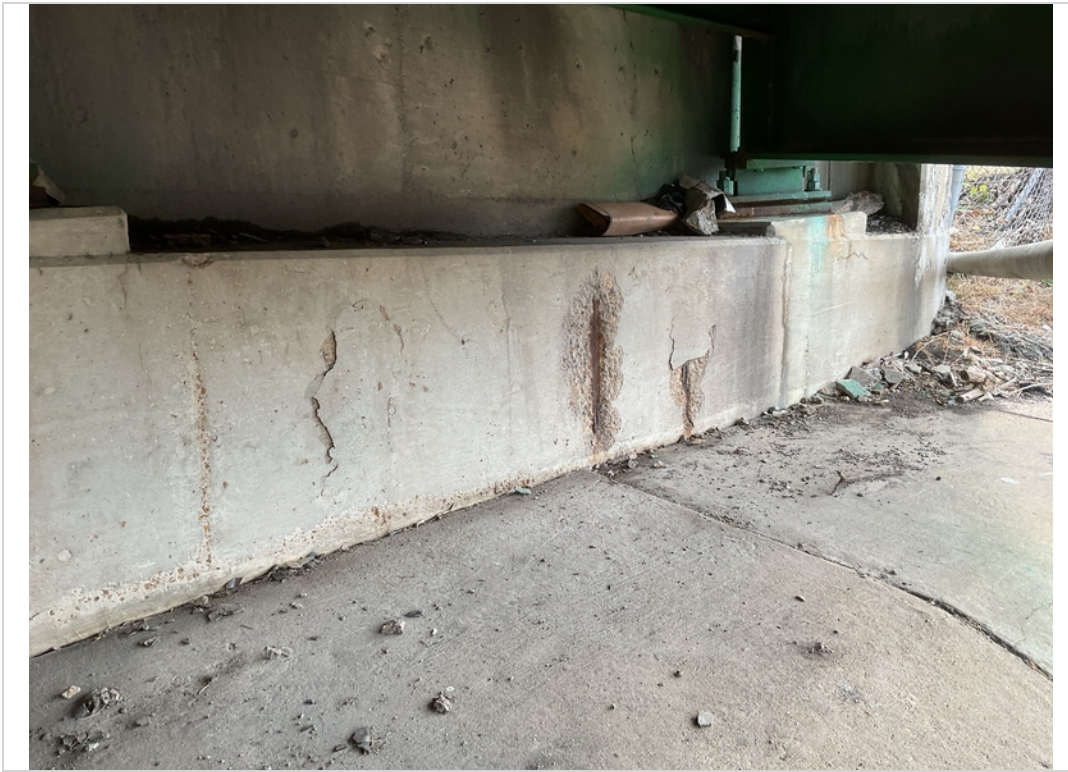
Abut 2 areas of delam w/exp steel
