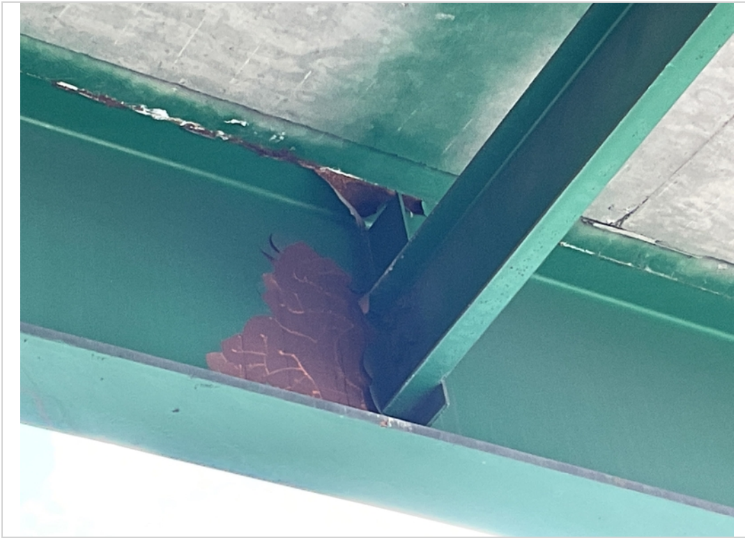
Span 2 Girder A corrosion
