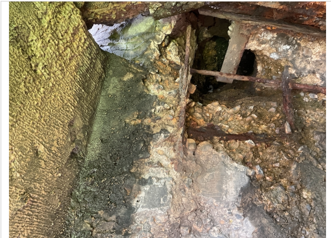
Abut 1 right spall w/exp steel
