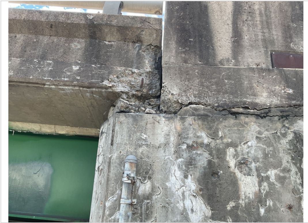
Abut 1 left spill w/exp steel on parapet
