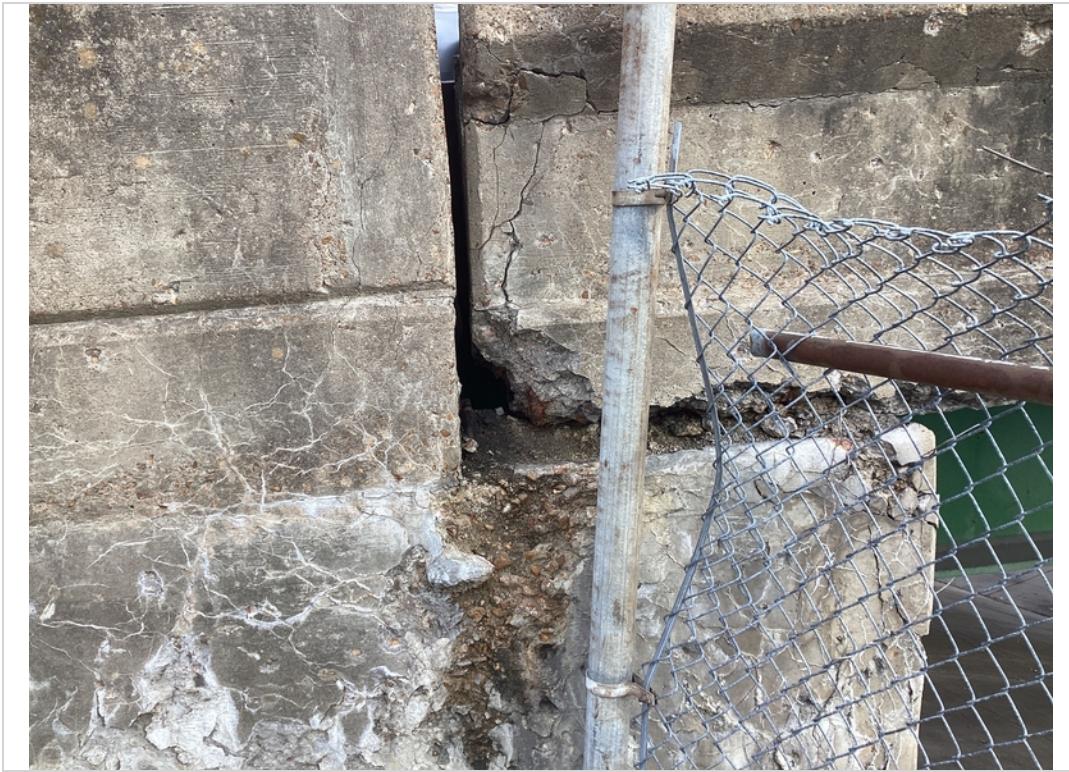
Span 1 parapet at right wing cracks spalls with exposed steel
