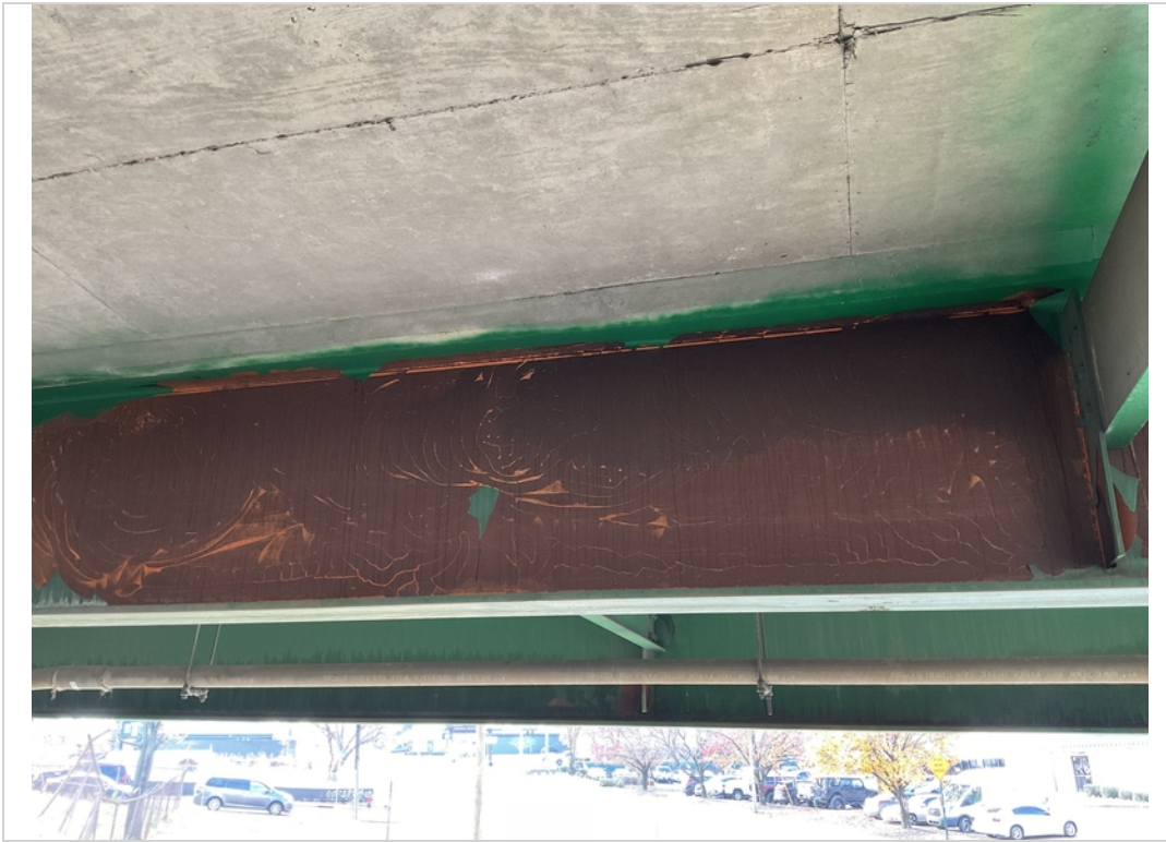
Span 3 Girder D corrosion
