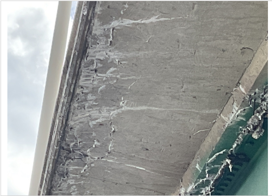
Overhang span 1 left side map cracks with eff
