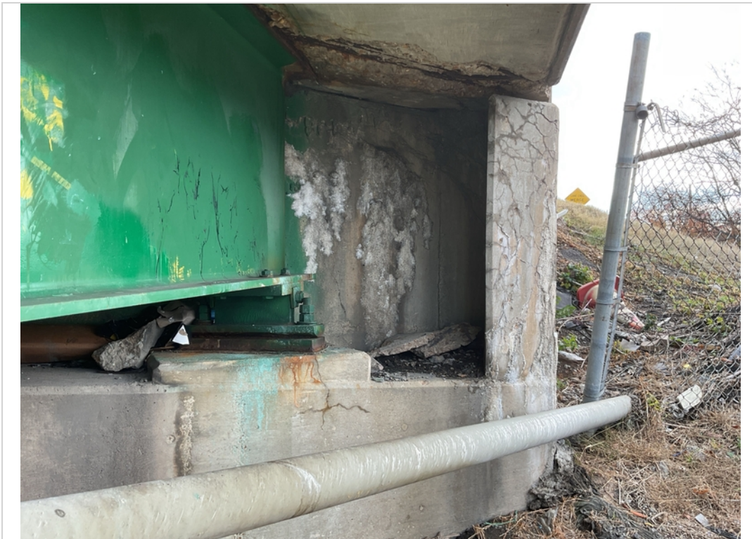
Abut 2 map cracks w/hvy eff
