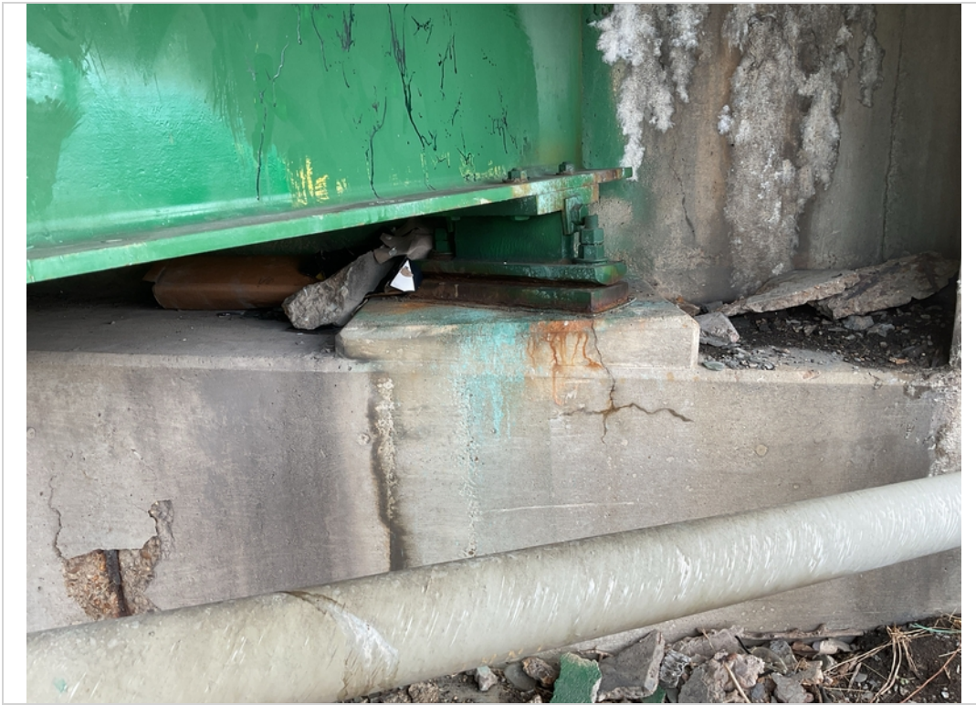
Abut 2 bearings moderate corrosion and debris
