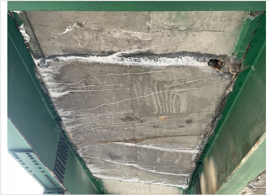
Span 1 bay A failing patch will eff
