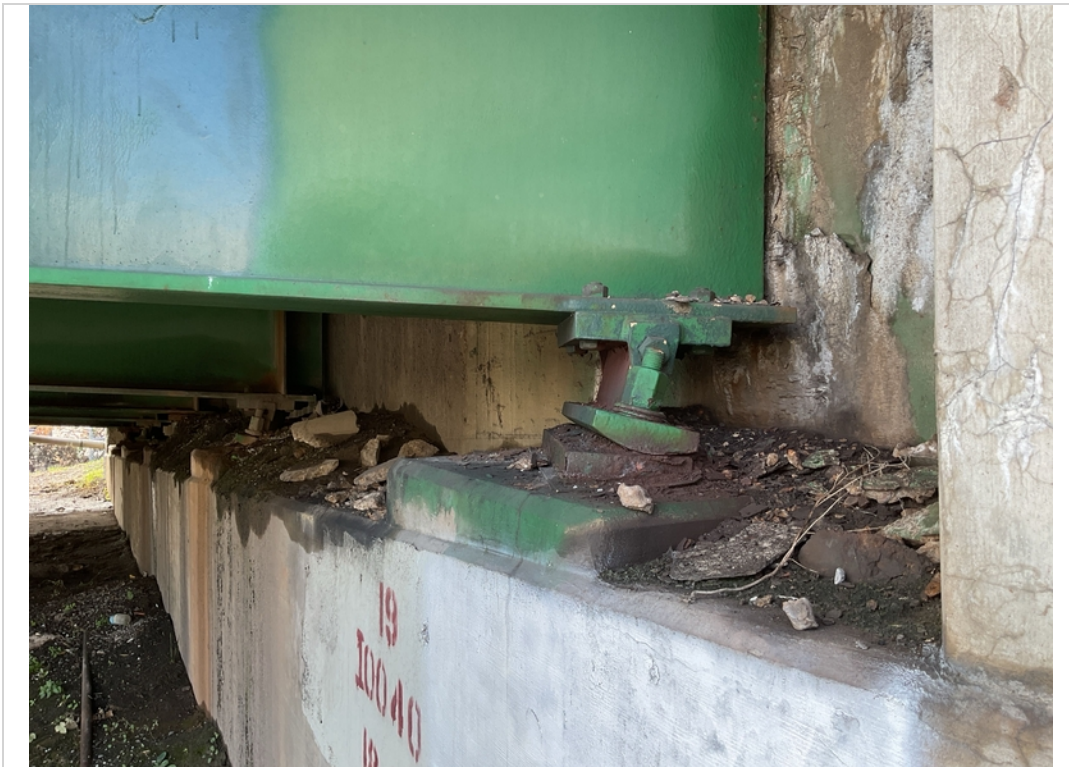
Abut 1 all bearings rocked back w/hvy debris build up.
