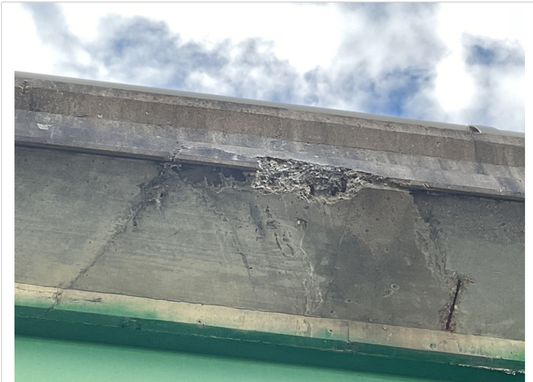
Overhang span 2 left side scale with exp steel
