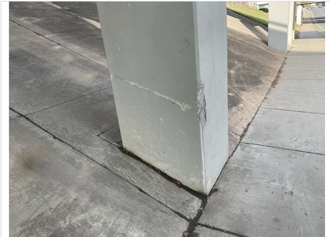
Pier 1 column A impact damage.
