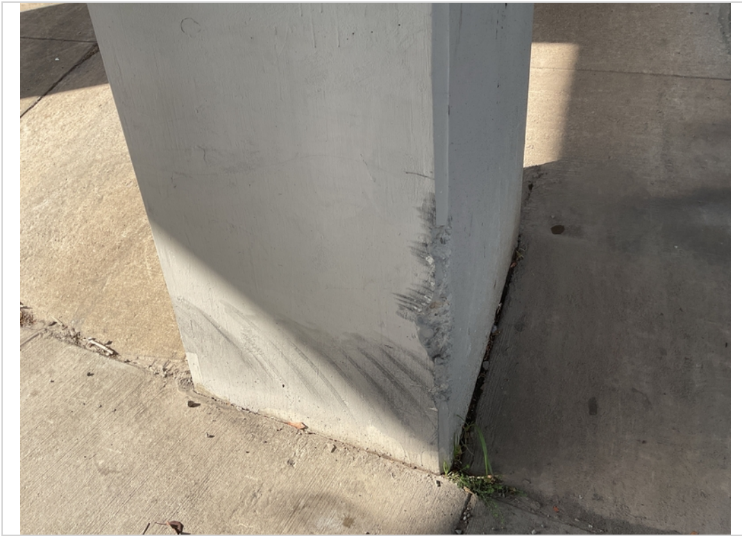
Pier 1 column B impact damage
