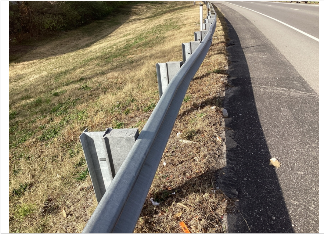
A approach guardrail impact damage
