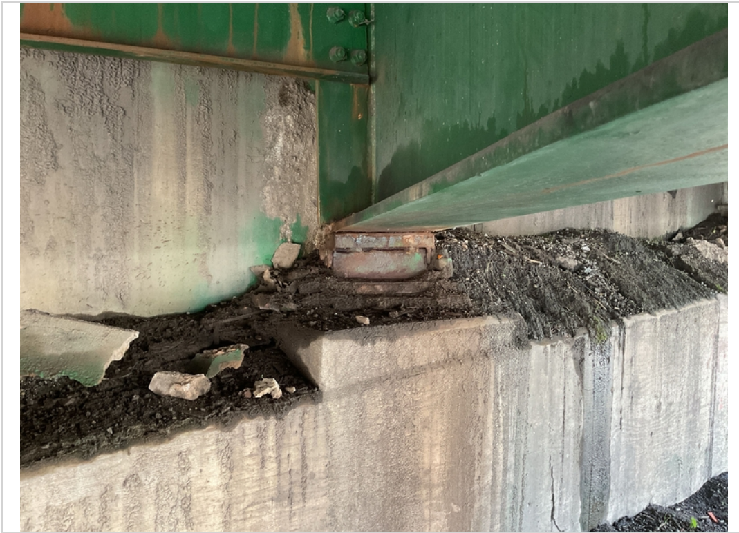
Abut 1 bearing C hvy corrosion loose or missing anchorage hvy build up
