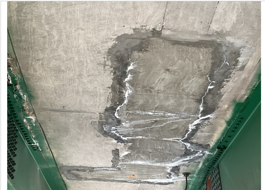
Span 1 bay B failing patch with eff
