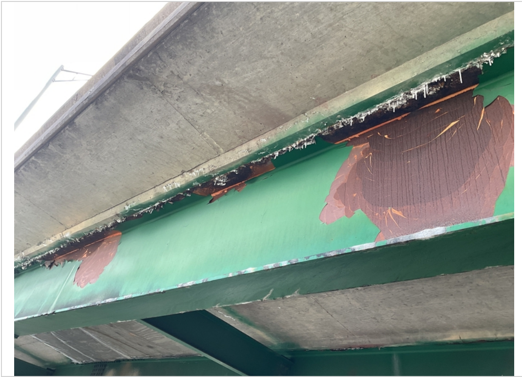
Span 1 Girder A top flange corrosion with eff
