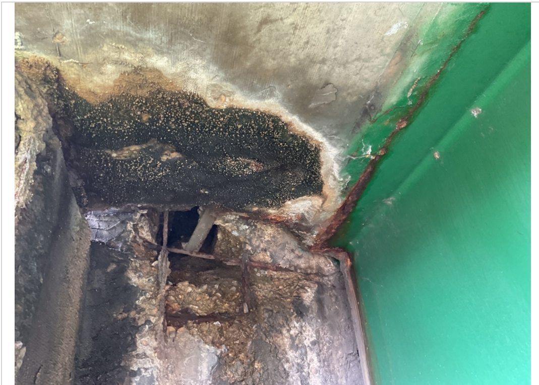
Overhang span 1 right side spall with eff
