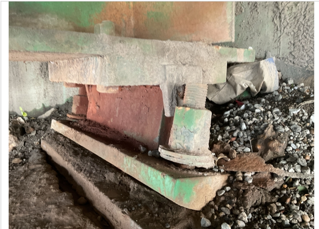
Abut 1 Bearing B broke pin loose anchorage
