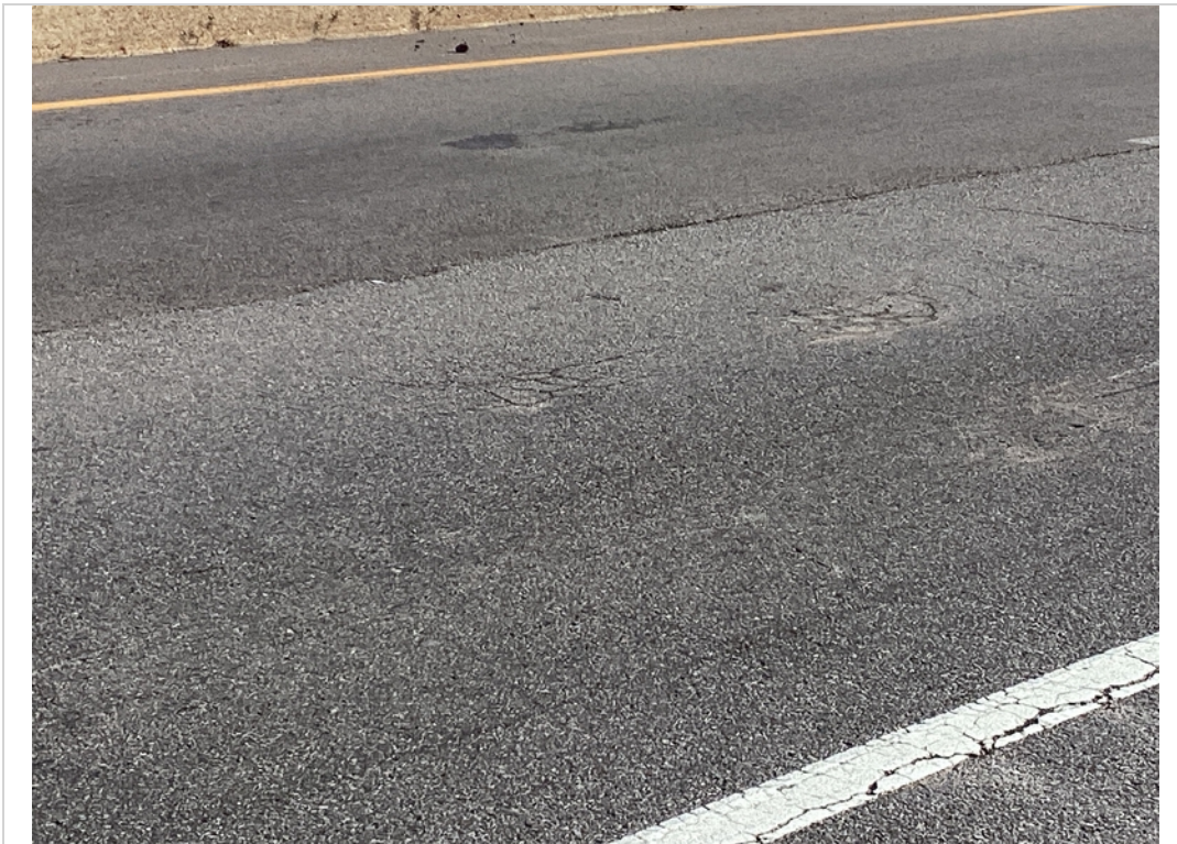
Span 1 depression with map cracks
