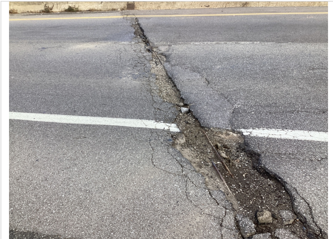
Span 1 joint paved over with potholes
