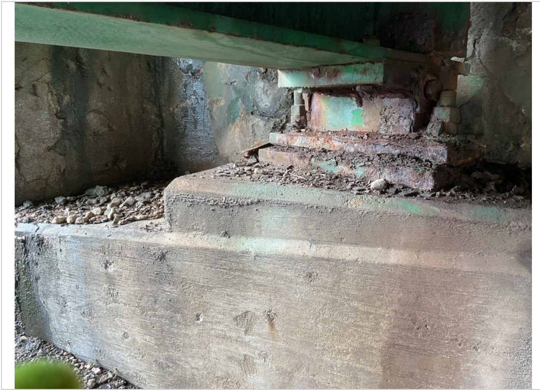
Abut 1 bearing E hvy corrosion loose or bent anchorage
