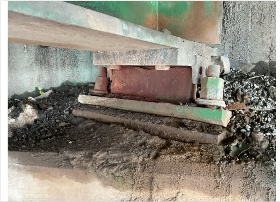
Abut 1 all bearings hvy corrosion w/ loose or missing anchorage
