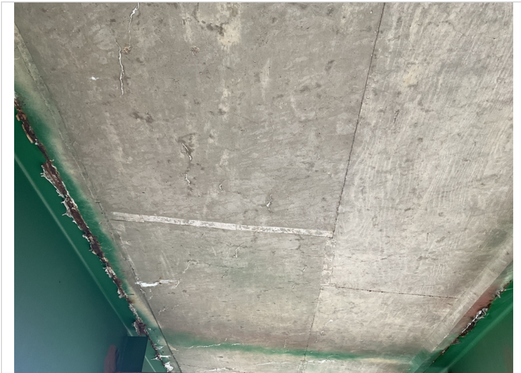
Span 1 bay A random map cracks with eff
