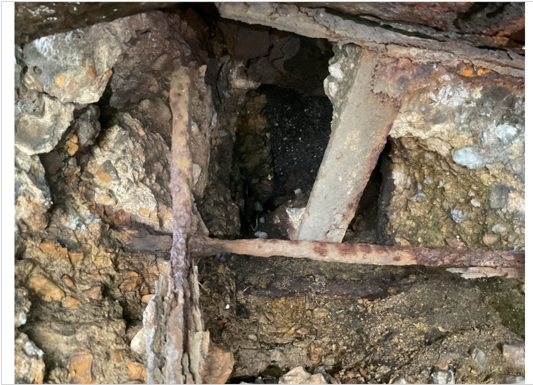
Abut 1 right back wall void w/exp steel exposing underside of wearing surface
