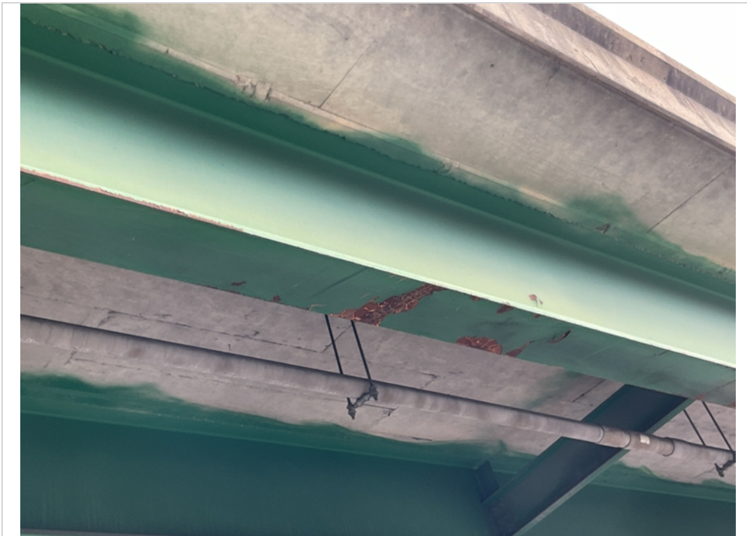
Span 2 Girder E impact scrapes
