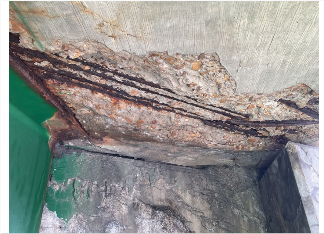
Overhang span 3 right side spall with exp steel
