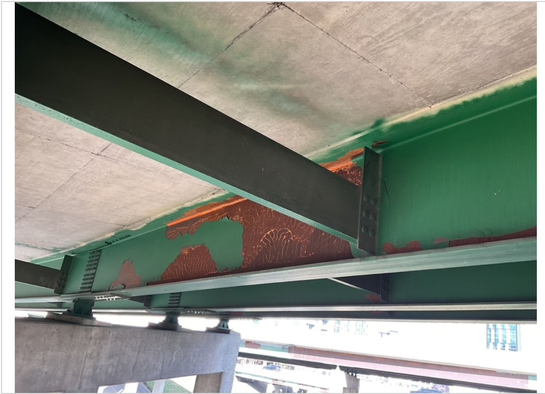
Span 3 Girder C corrosion
