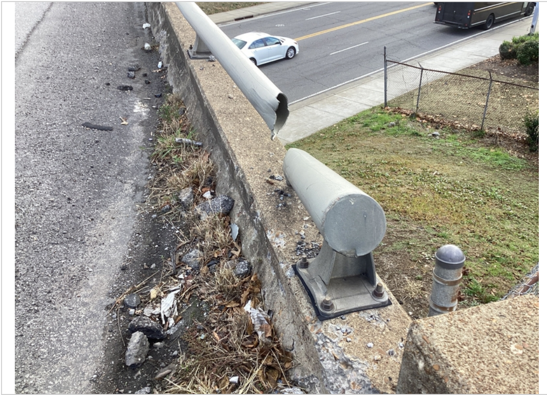
Span 1 tube rail broken
